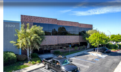
2820-2834 La Mirada Drive 5,520 SF - 22,914 SF - Manufacturing $1.49 - $1.55 MG/PSF
