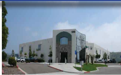
3280 Corporate View 59,828 SF - Warehouse $1.05/NNN
