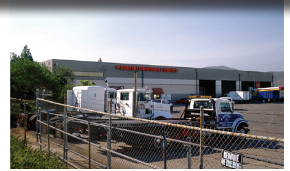
160 Industrial St. 18,400 SF - Service $1.05/NNN
