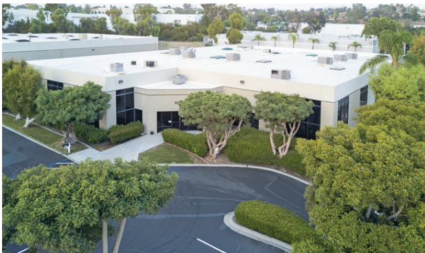
2636 Vista Pacific Dr. 21,260 SF - Warehouse $3,656,000 ($171.97/PSF)
