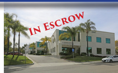
2067 Wineridge Pl., Unit D 35,550 SF - Warehouse $1,197,795 ($235.00/PSF)
